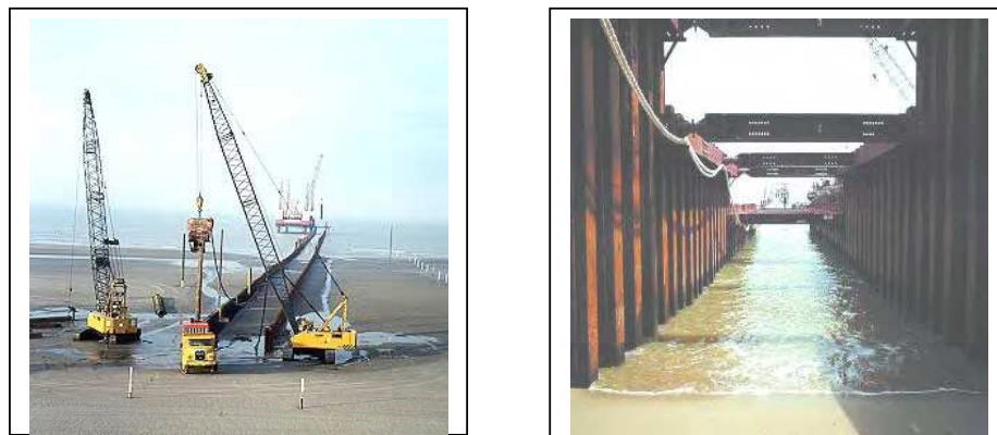
Figure 3.10 Illustration of a Typical Cofferdam Construction
