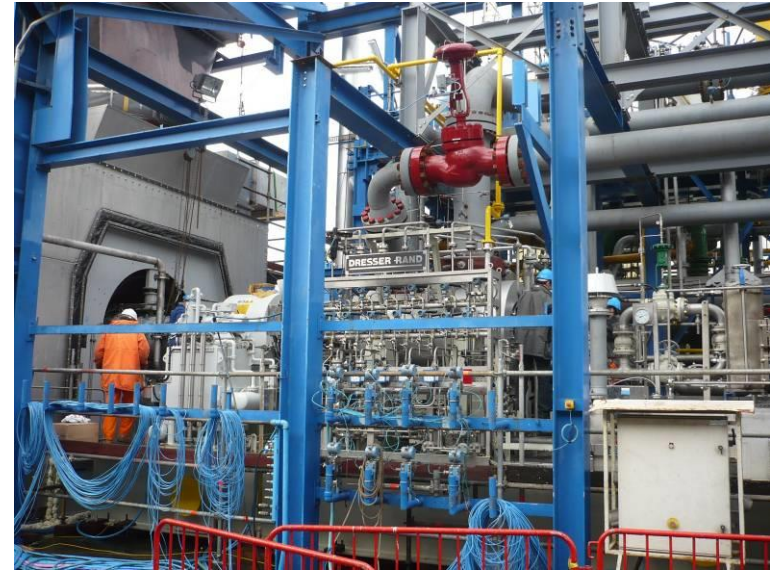
➤ Turbocompressor preparation. Le Havre, February 2008
