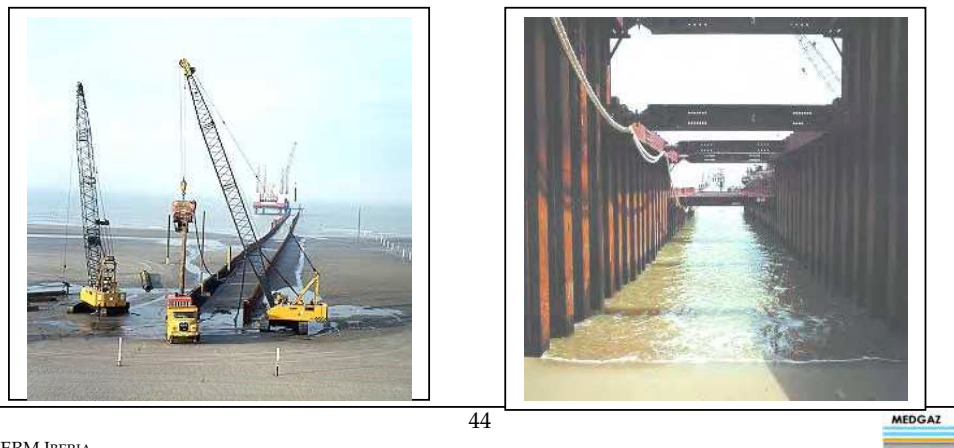
Figure 3.10 Illustration of a Typical Cofferdam Construction
